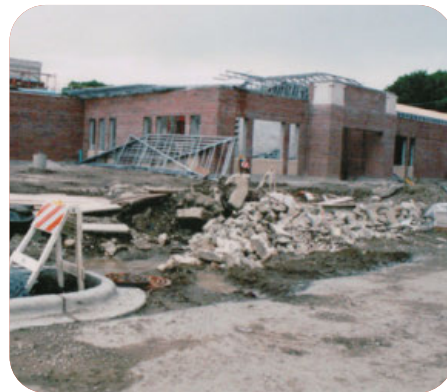
The Construction Zone
